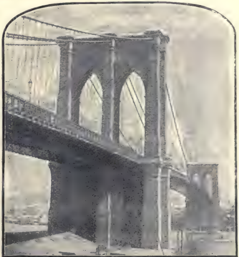
FIG. 158—Brooklyn Bridge, New York
